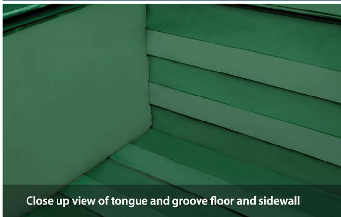
Close up view of tongue and groove floor and sidewall
